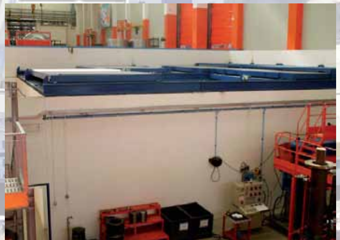
Our Bunker at Valvitalia plant
